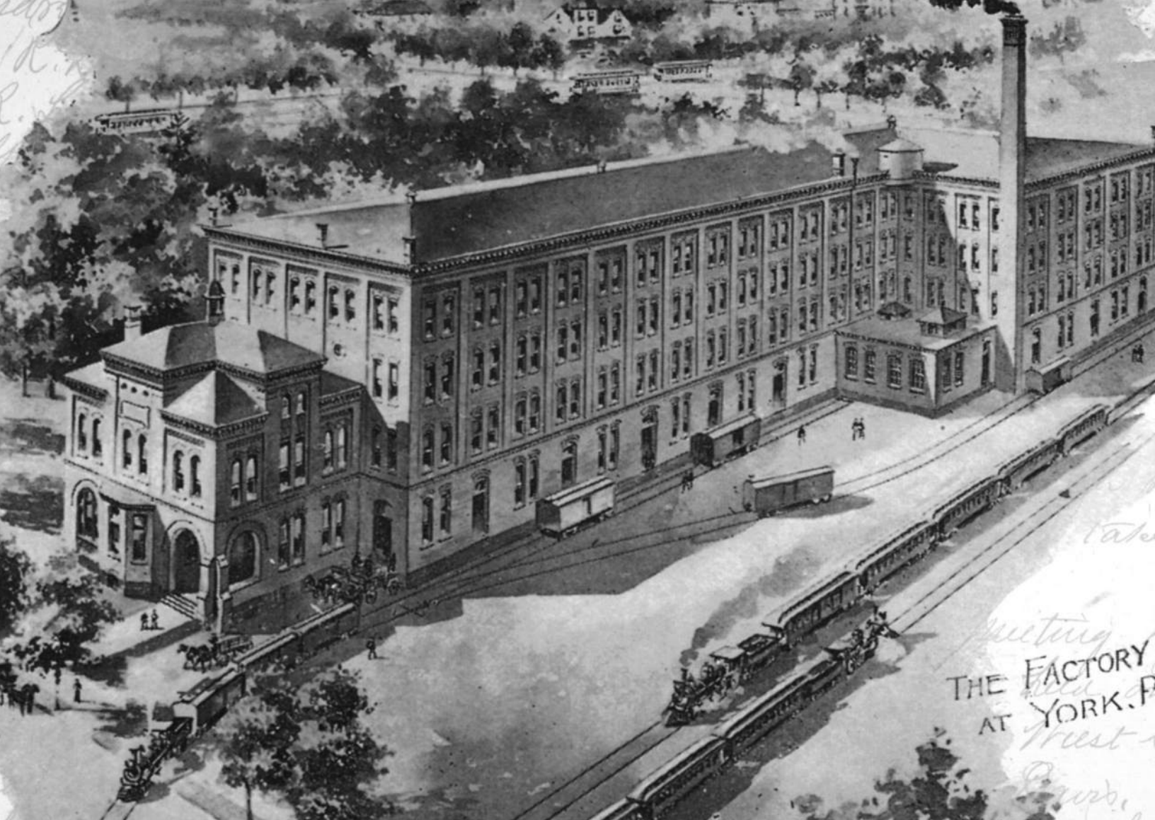
York Wallcoverings Factory 1900s
