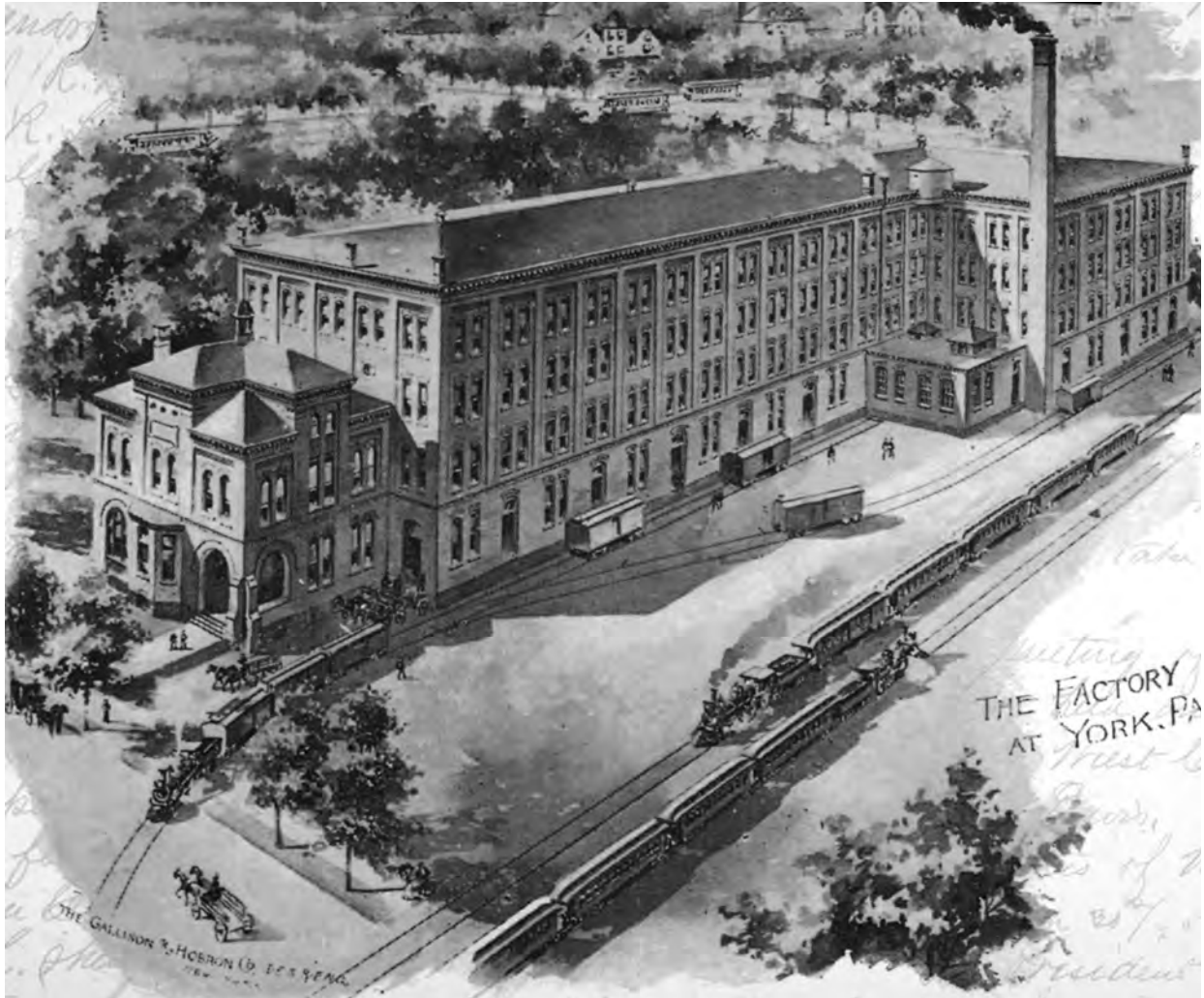
York Wallcoverings Factory 1900's
