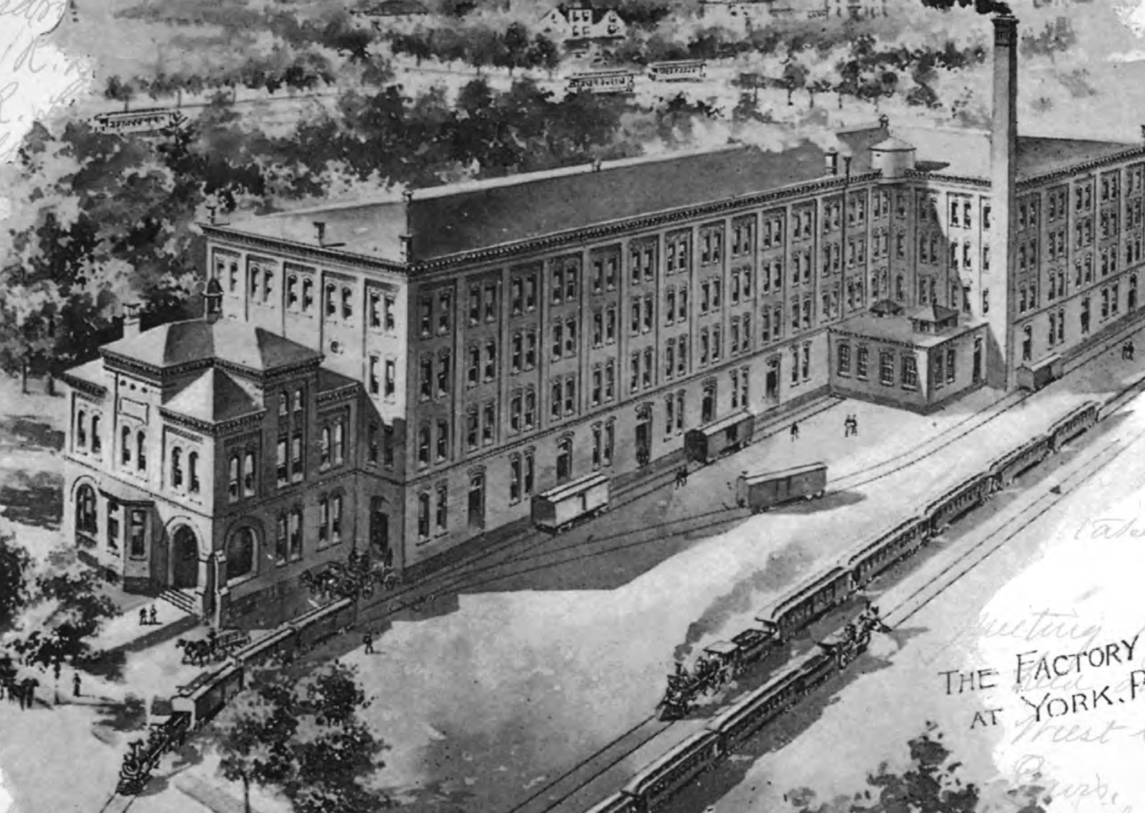
York Wallcoverings Factory 1900s
